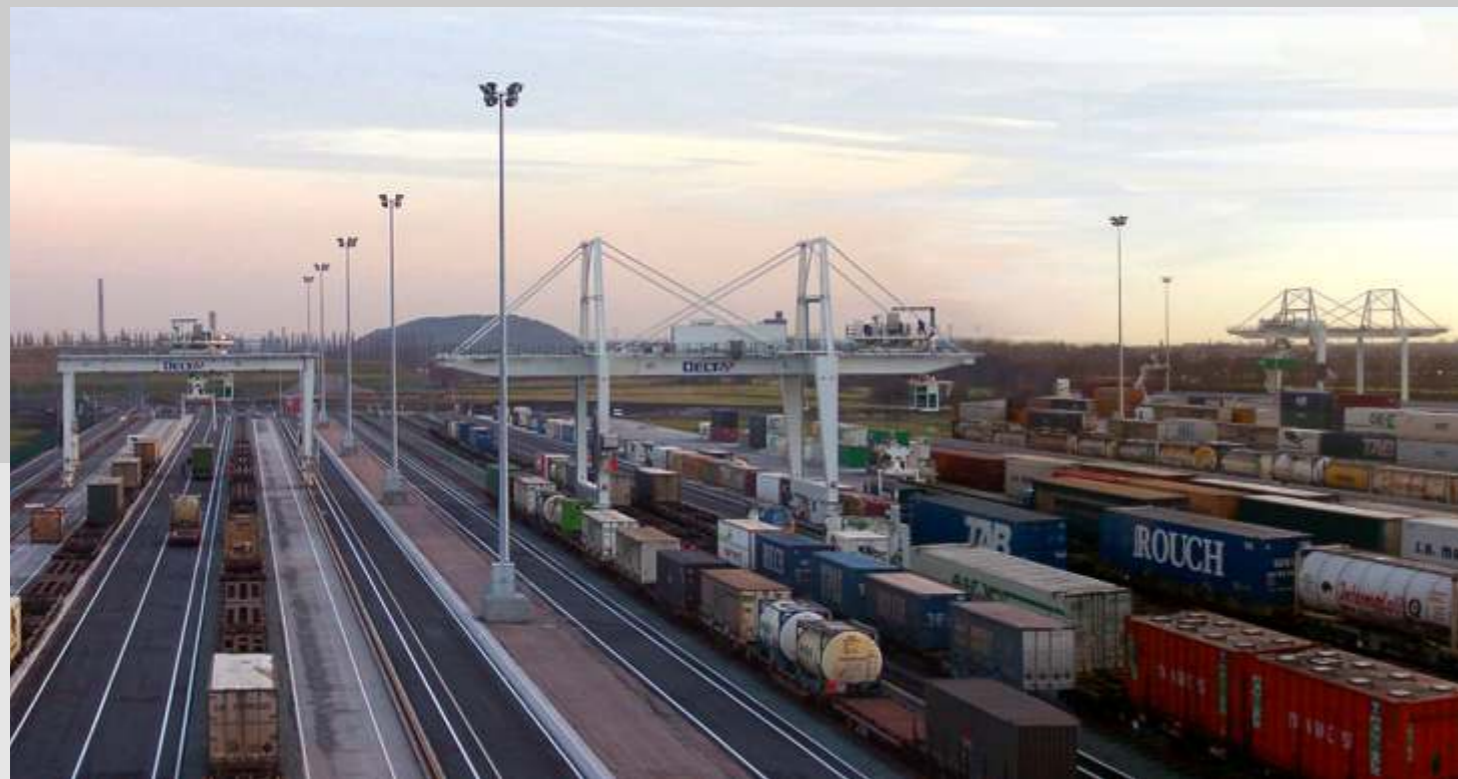
5 container RMG cranes for Terminal Delta-3 in river port Dourges, France
