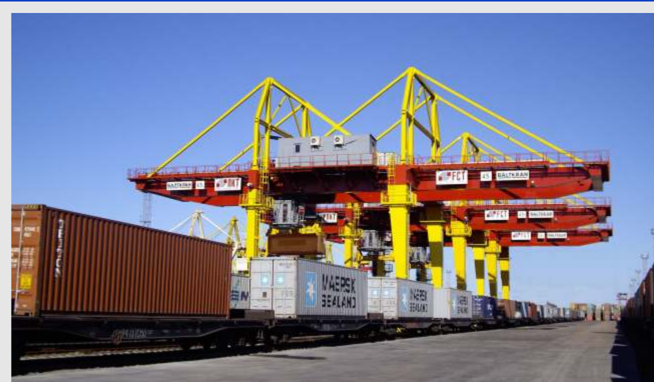
CONTAINER RAIL MOUNTED GANTRY CRANES
